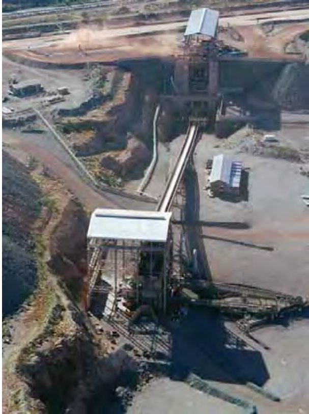
Sishen Expansion Project, South Africa.
